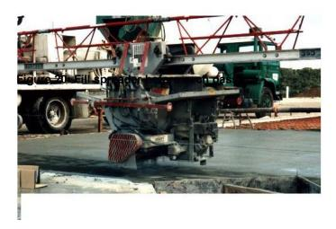
Figure 21: Spreader applying the shake
