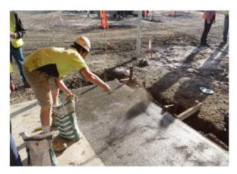
Figure 5: Allow the shake to fall onto the surface from above
