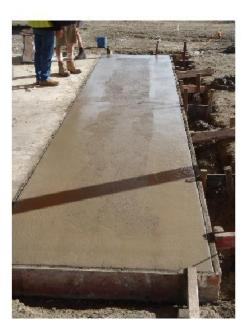
Figure 2: Screeded concrete prior to application of the shake
