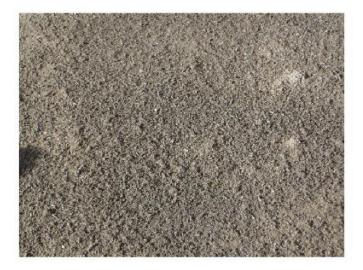
Figure 10: shake prior to trowelling notice the colour is uniformly dark.
