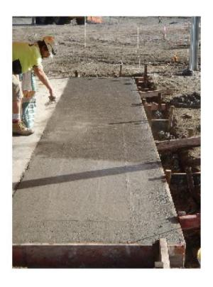
Figure 4: See how the shake soaks up the moisture from the fresh concrete
