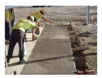
Figure 6: Ensure that the correct amount is applied per square meter.
