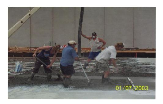
Figure 18: Apply shake directly behind the screed
