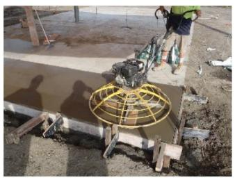
Figure 14: Keep the blades flat to consolidate the shake
