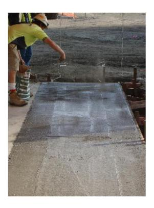
Figure 3: Applying the shake into the freshly screeded concrete
