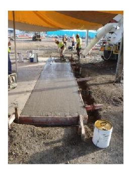
Figure 1: Screeding the concrete
