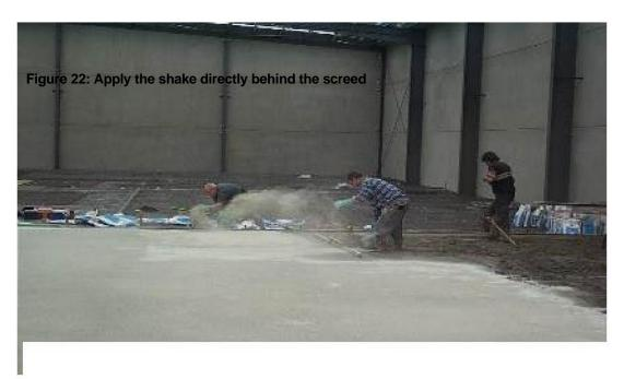
Figure 23: Applying the shake in the "feeding the Chooks " method
