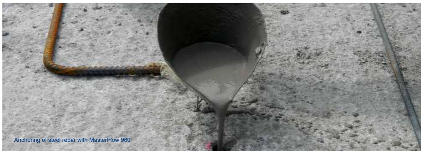
Anchoring of steel rebar with MasterFlow 960
