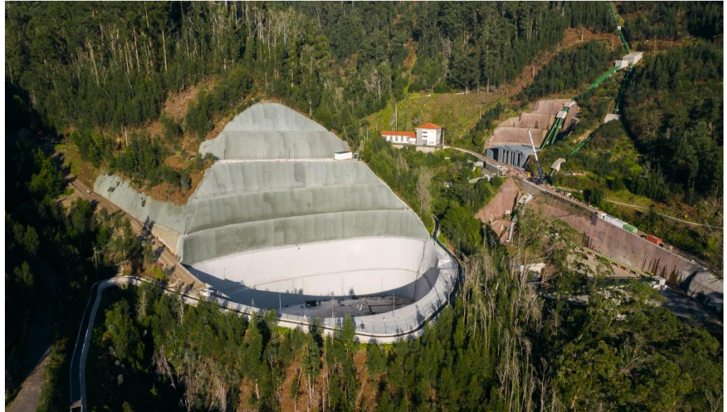
Our reference project at Madeira, Portugal: Waterproofing of the buffer reservoir in the Calheta hydroelectric power plant.
