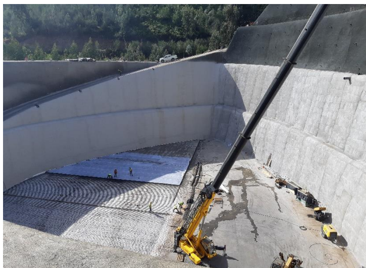
Our reference project at Madeira, Portugal: Waterproofing of buffer reservoir in the Calheta hydroelectric power plant.
