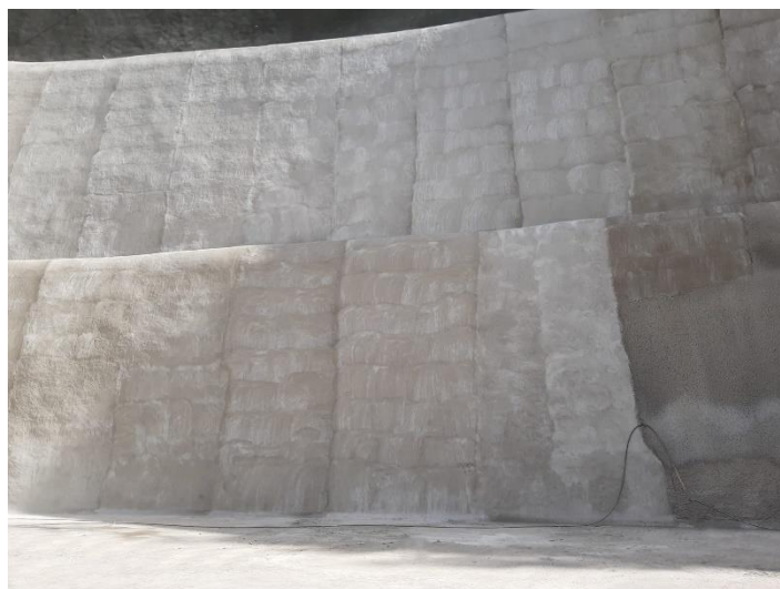
Our reference project at Madeira, Portugal: Waterproofing of buffer reservoir in the Calheta hydroelectric power plant.
