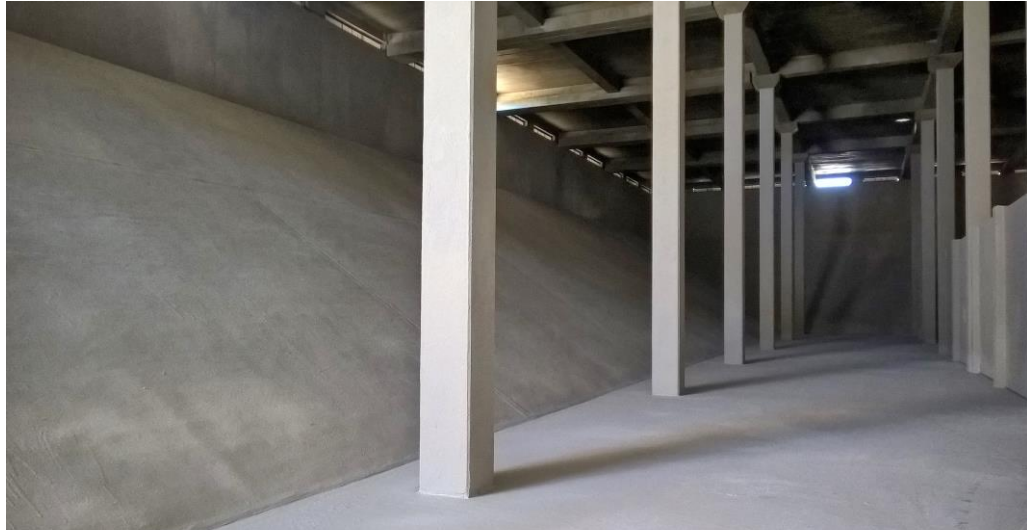
Our reference project in Granada (Spain): Loaysa Water Tank
