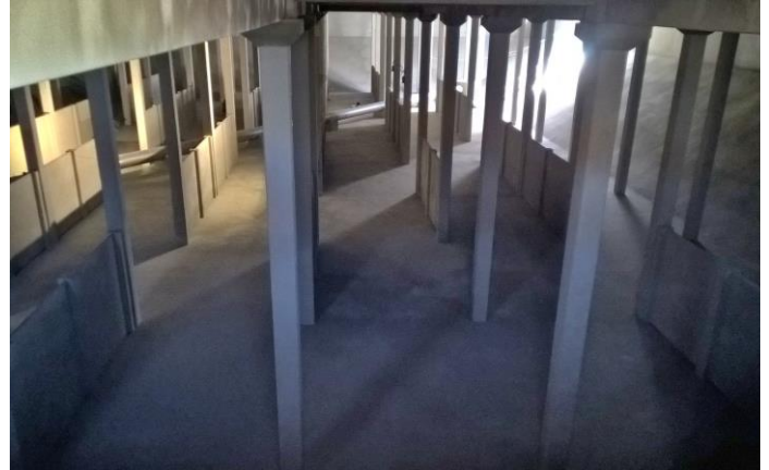
Our reference project in Granada (Spain): Loaysa Water Tank
