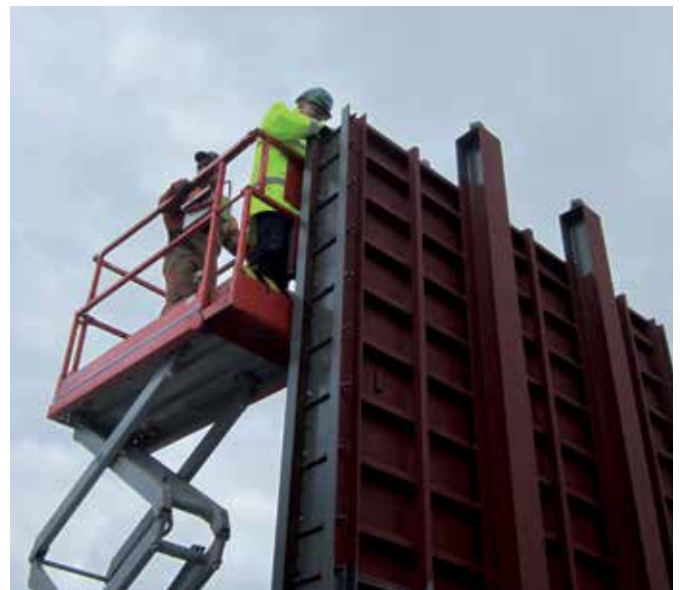
Industry expert inspecting grouting mock-up
