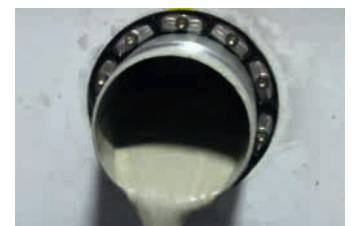
Bolted connection and grout overflow
