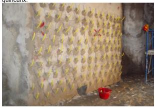
In correspondence of each hole, an injection tube with a diameter of 15 ÷ 20 mm is inserted to a depth of about 10 cm. The injector is fixed and seals perfectly.
