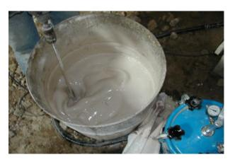
To obtain a perfect mixing it is advisable to initially add only part of the mixing water to the powder product and to homogenize at low speed for a few minutes, then add the remaining part of water necessary to obtain the desired fluidity, stirring for a few more minute until a fluid, homogeneous and lump-free mixture is obtained.
