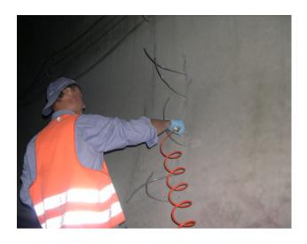
Eliminate the crumbly and incoherent parts and carefully dust the surface with compressed air, then attach copper tubes with a section of 8 mm in the holes, seal the cracks and fix the injection tubes with the adhesive MasterBrace ADH 4000.
