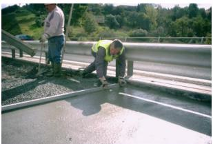
Casting into formwork of the mortar is continuous and from one side only to avoid air entrapment.
