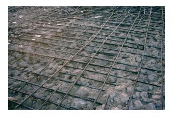
Loose or contaminated concrete must be removed preferably by hydro demolition or, alternatively, by mechanical chipping using lightweight compressed-air operated concrete breakers and taking all the necessary precautions to avoid damaging the structures.
