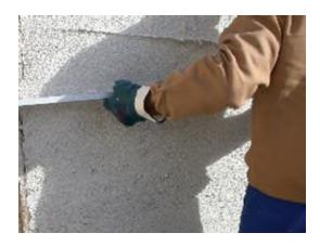
once the required consistency has been reached, float the surface with a wet sponge float;
