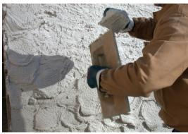
level with an aluminium straight edge with a knife profile;
