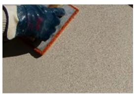
if the maximum thickness of 3-3.5 cm is to be applied, once hardened and roughened and moistened with water, subsequent coats must be applied at a thickness not exceeding 1-1.5 cm.
