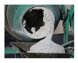
after hardening of the rough coat on the damp substrate, apply a 1.5-2 cm macro-porous layer of plaster by trowel;
