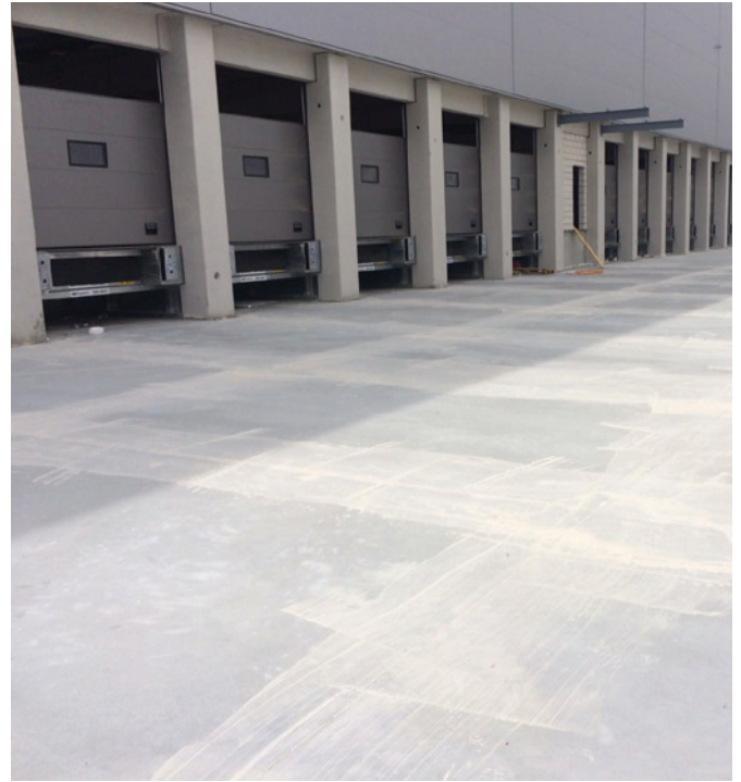
MasterFiber Pavimento industrial, Madrid
