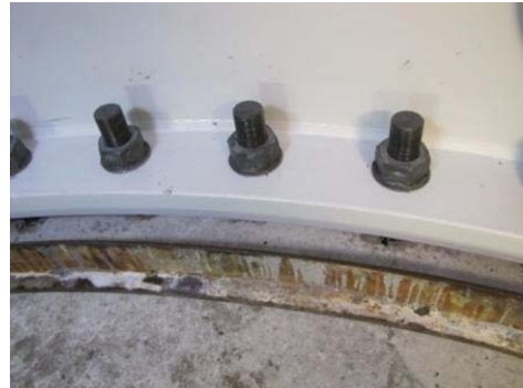
Steel formwork installed on the inside
