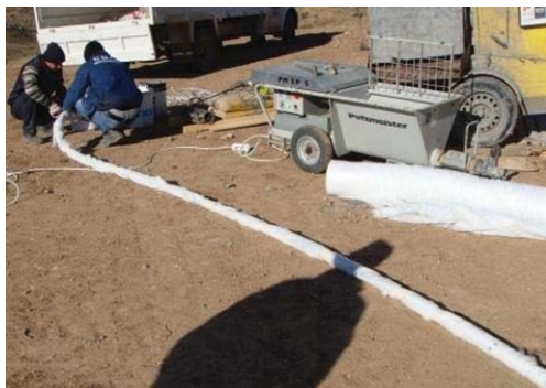
Reflective installation being applied to the hoses
