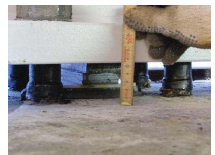
Situation showing tower base installed on shims
