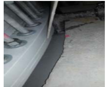
Pumping Masterflow 9400 underneath the flange of the tower
