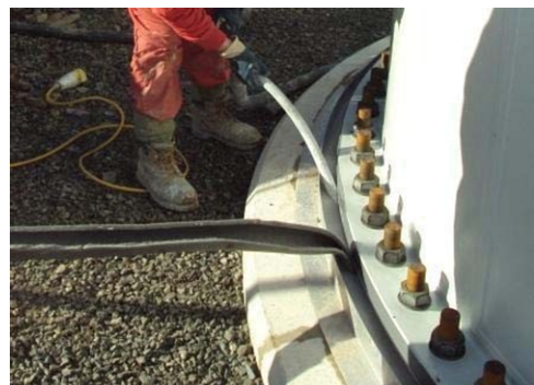
PU-foam used as temporary form
