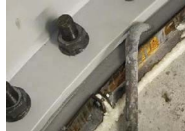
Rigid thin wall metal tube to pump underneath flange
