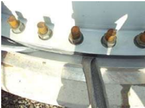
PU-foam used as temporary form
