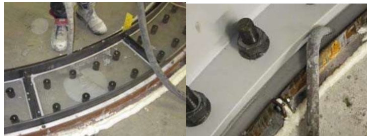
Rigid thin wall metal tube to pump underneath flange
