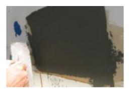
3. For the base coat, embed a 4" wide strip of Flexguard 4 reinforcing mesh into wet material; for Senershield products embed 4" Sheathing Fabric into the wet material. Additional base coat or a Senershield air barrier can be applied to ensure full embedment. Use sufficient mesh or Sheathing Fabric so that 6" is embedded and 6" is left exposed for a pull tab.
