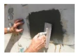
4. For base coats it is recommended to allow 48 hours cure time; for Senershield products 24 hours of dry time is recommended prior to pull
