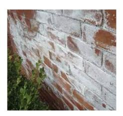
In most cases, power washing is effective in removing dust, dirt and environmental contaminants, however, use of efflorescence cleaning products may be necessary. Painted or sealed surfaces might require high-pressure power washing.
