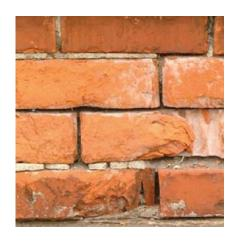
Deteriorated masonry will generally need some level of repair prior to over cladding with EIFS. When spalling has occurred, related problems such as water damage might have already affected the interior of the wall in some way. Always consult with a structural engineer who can develop an assessment of the building that includes a thorough evaluation of any damage.
