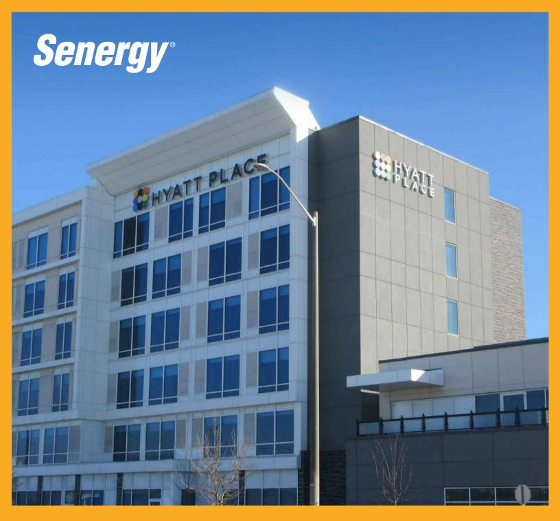
Water Drainage Class PB Exterior Insulation and Finish System Using Mineral Wool Insulation
