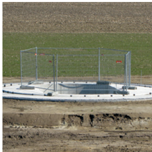
Concrete tower foundation
