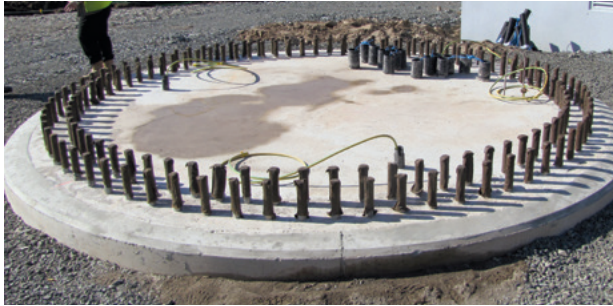
Concrete foundation ready to install turbine
