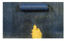
**3.** Apply a first layer of MasterBrace SAT 4500 or 4700 using a 3/8" nap roller.
