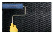
5. Set the dry fiber fabric into wet saturant and press to the surface using a rib (defoaming) roller. Apply a second layer of saturant to fully encapsulate fibers. Repeat saturant/fiber/saturant layers as nedeed.
