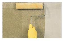
**1.** Apply MasterBrace P3500 using a 3/8" nap roller.
