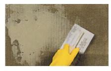
Apply MasterBrace F2000 using a trowel or putty knife to level uneven surfaces.
