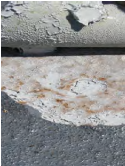
D. Improper mixing
