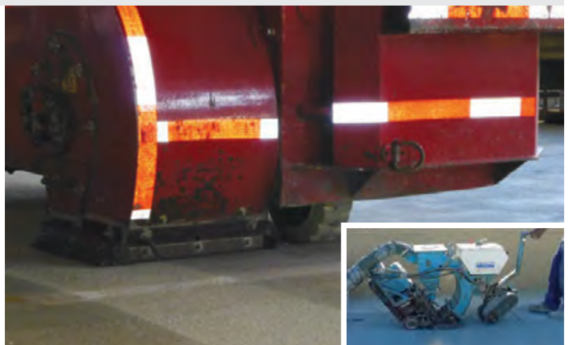
Shotblasting a concrete substrate
