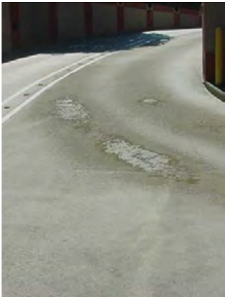
D. Incorrect System Selection
