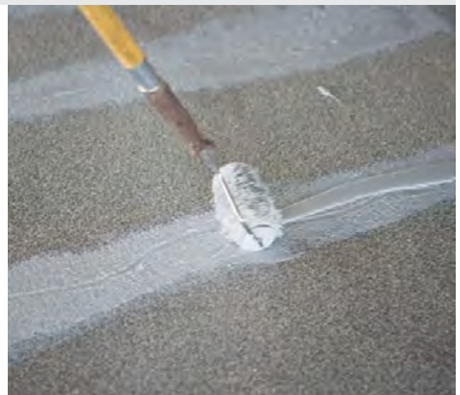
Detailing cracks
