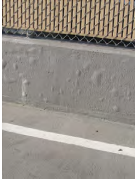
B. Excessive vapor drive
