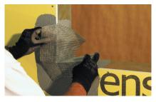
Step 3: Place MasterSeal® AWB 975 FIB on the MasterSeal® AWB 660/MasterSeal® AWB 665/ or MasterSeal® AWB 660 I material
