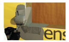
Step 4: Completely satuarate MasterSeal® AWB 975 FIB with MasterSeal® AWB 660/MasterSeal® AWB 665/or MasterSeal® AWB 660 I material
