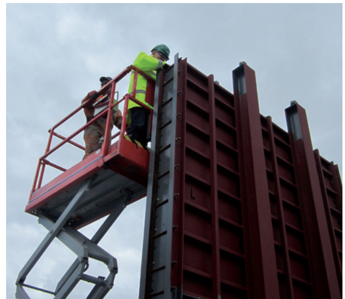
Industry expert inspecting grouting mock-up
