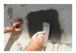
4. For base coats it is recommended to allow 48 hours cure time; for Finestop products 24 hours of dry time is recommended prior to pull
