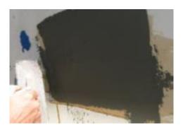
3. For the base coat, embed a 4" wide strip of Finestone reinforcing mesh into wet material; for Finestop products embed 4" Sheathing Fabric into the wet material. Additional base coat or a Finestop air barrier can be applied to ensure full embedment. Use sufficient mesh or Sheathing Fabric so that 6" is embedded and 6" is left exposed for a pull tab.
