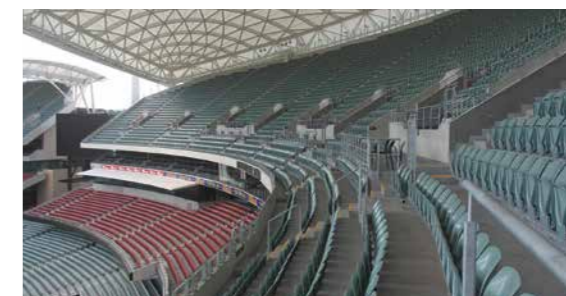
MasterSeal Traffic 2000 HD Adelaide Oval grandstand, Australia
