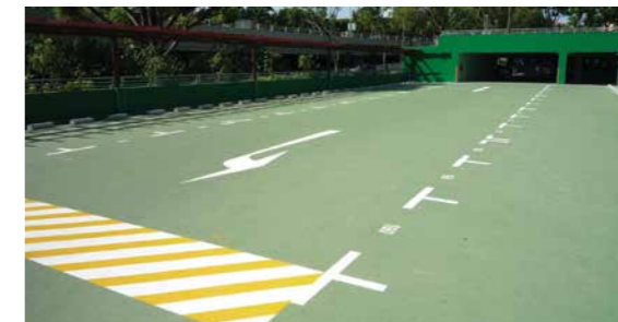
MasterSeal Traffic 2500 HD MacRitchie reservoir car park, Singapore
