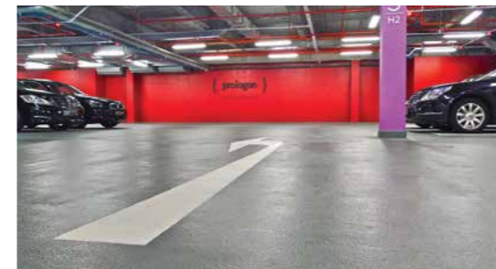
MasterSeal Traffic 2500 HD Ion Orchard car park, Singapore
