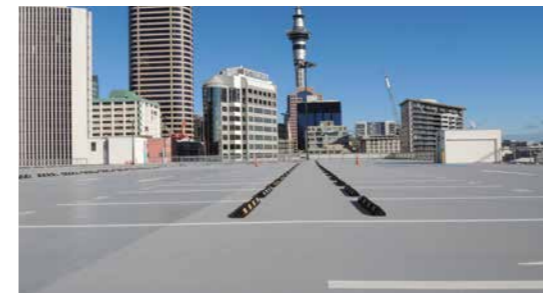
MasterSeal Traffic 2000 HD Auckland downtown car park, New Zealand
