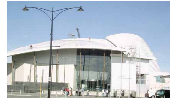
MasterSeal Roof 3500 Maritime Museum, Western Australia
