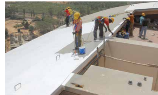
MasterSeal Roof 3500 Brigade condominium, India
