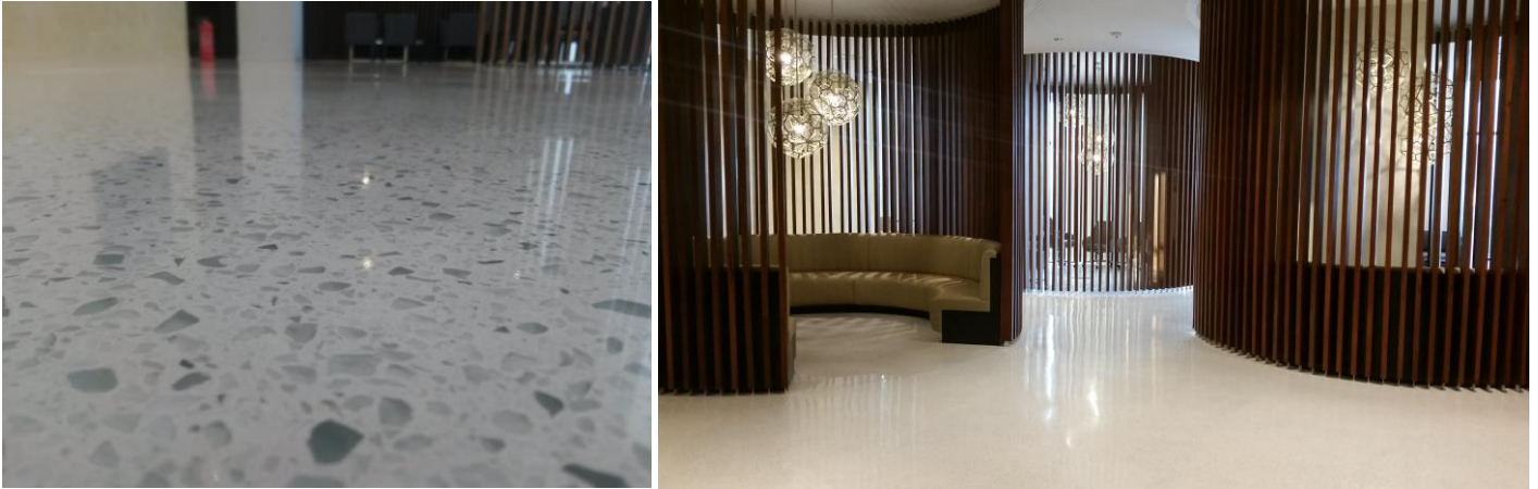
Our reference in Al-Khobar, Eastern Region (Kingdom of Saudi Arabia): Staybridge Suites Project Pictures Source: visit to the site.
