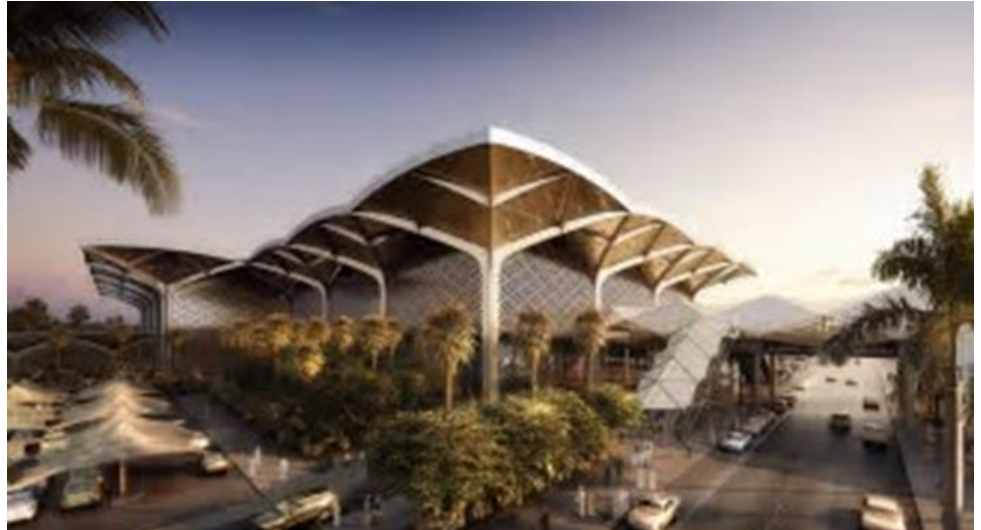
Our reference in western province (Kingdom of Saudi Arabia): Haramain High Speed Railway Stations Picture Source: Google Maps.
