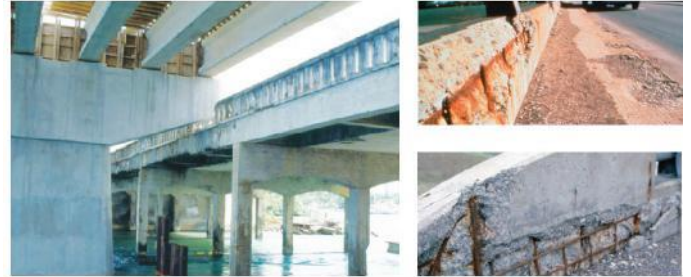
The bridge on the right is experiencing heavy corrosion. The bridge on the left was built to prevent corrosion by using high performance concrete with durability-enhancing admixtures. Durability issues, such as corrosion of reinforcing steel in roads, bridges, and parking structures, can be effectively addressed with durability-enhancing admixtures from Master Builders Solutions.
