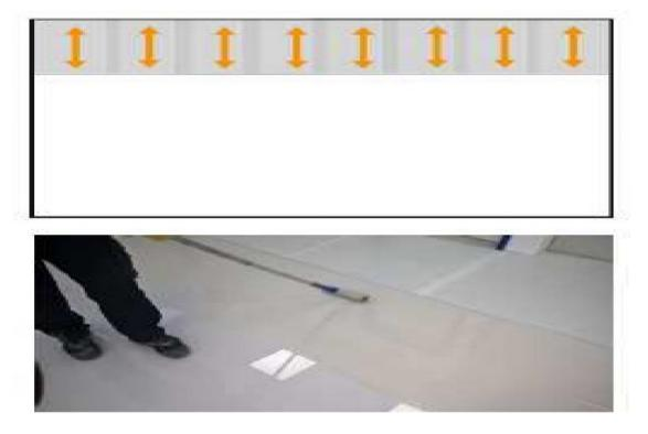
Application with the squeegee must continue whilst step 2 is in progress to ensure a wet edge is maintained. In areas with difficult geometry in may be necessary to stand in the wet material while conducting step 2. In this case either use rounded spike shoes or protect the sole of shoes with sandpaper (see step 3).
