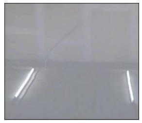
To remove air bubbles, spike-roll the surface after application and depending on jobsite conditions. Make sure that the surface looks good, smooth, well leveled and without any defects like "fish eyes", "pin holes", air bubbles or dirt & impurities:
