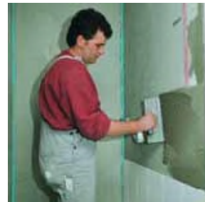
6. When the waterproofing MasterTile WP 668 has cured tiles can be laid.
