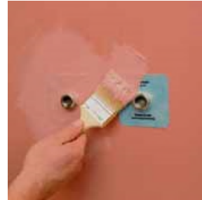
4. Place MasterTile WP Tape over the pipe connection protruding from the wall and cover with MasterTile WP 668 (red)
