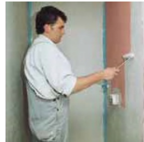
5. After an evaporation time of approx. 1 hour apply the second protective coating with MasterTile WP 668 (grey). The first coat of MasterTile WP 668 (red) should not be visible, otherwise another layer might be necessary.
