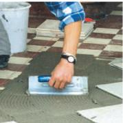
Subsequent top coverings can be applied after approx. 30 to 45 minutes using MasterTile tile adhesives
