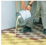
2. Shake **MasterTile P 303** well before use and pour onto the substrate.
