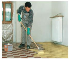
**MasterTile P 303** is the reliable primer for laying coverings on ceramic tiles and flagstones.
