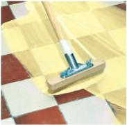
3. Spread primer over the substrate working in criss-cross method
