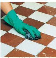
Use a suitable cleaning agent to remove residues which could impair adhesion from the substrate
