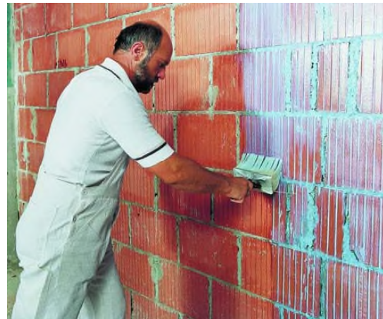
MasterTile P 302 helps improve adhesion of plaster and lime plastering to brickwork.
