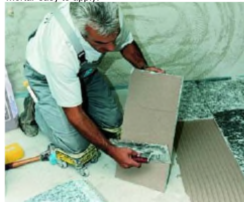
For void-free laying always apply a layer of mortar to the reverse side of the tile.
