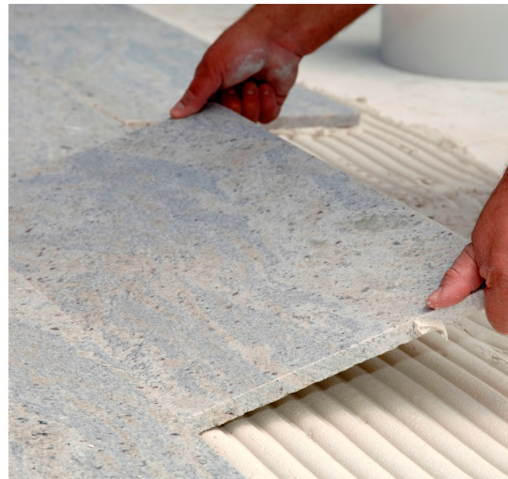
For void-free laying always apply a layer of mortar to the reverse side of the tile.
