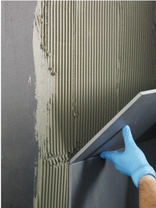
Secure laying of tiles with MasterTile FLX 420 .
