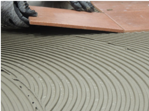
Secure laying of tiles with MasterTile FLX 23E
