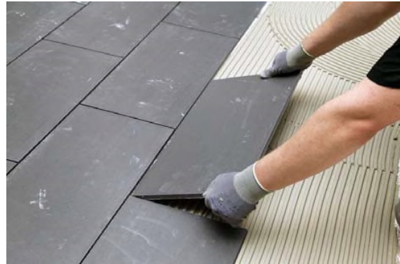
Secure laying of tiles with MasterTile 434
