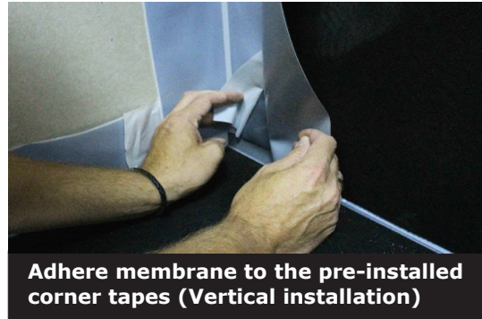
Adhere membrane to the pre-installed corner tapes (Vertical installation)
