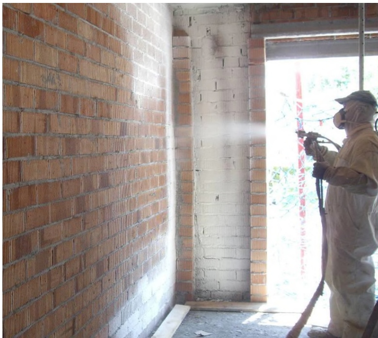
Application of primer layer over a ceramic substrate
