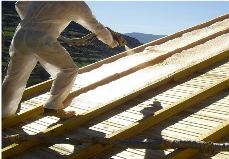
Application of the foam between rafters in a wood roof
