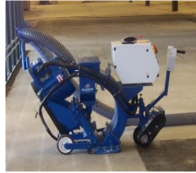
Mechanical preparation for the substrate, Blast Cleaning
