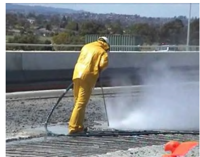
High pressure water blasting
