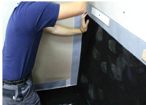
**Adhere membrane to the pre-installed corner tapes (Vertical installation)**
