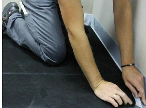
**Adhere membrane to the pre-installed corner tapes (Horizontal installation)**
