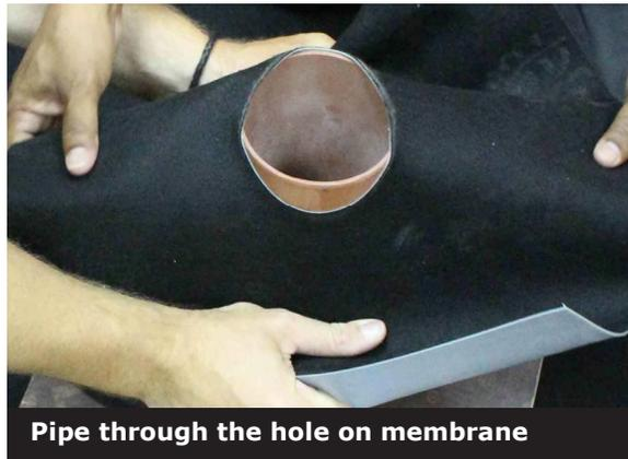
**Pipe through the hole on membrane**
