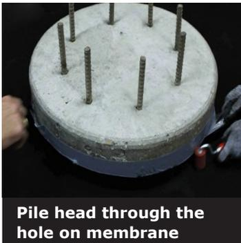
Pile head through the hole on membrane
