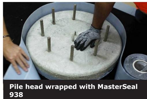
Pile head wrapped with MasterSeal 938
