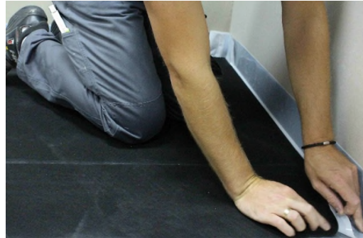
Adhere membrane to the pre-installed corner tapes (Horizontal installation)
