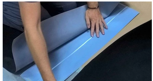
Butt-jointing with self-adhesive tape
