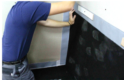
Adhere membrane to the pre-installed corner tapes (Vertical installation)
