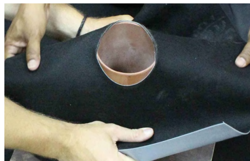
Pipe through the hole on membrane
