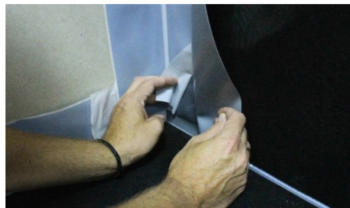
Adhere membrane to the pre-installed corner tapes (Vertical installation)
