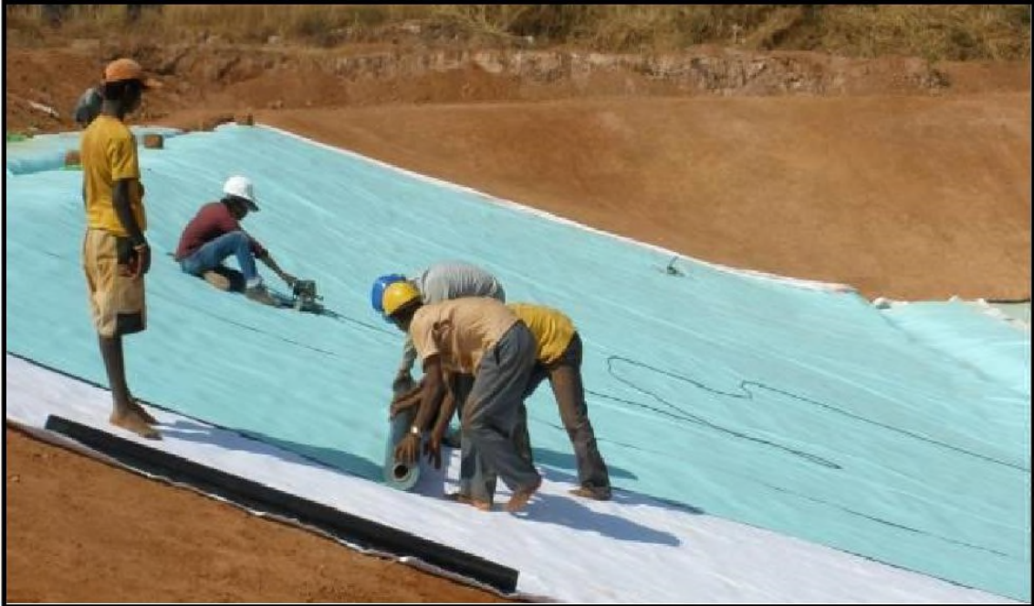
WATERPROOFING SYSTEM INSTALLATION
