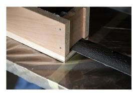
Using an "application box" as shown, apply a convex layer of MasterBrace ADH 4000 onto the pre-cleaned face of the MasterBrace LAM. The "gate" of the applicator box should be profiled to create a 2mm thick (in the centre) convex layer of MasterBrace ADH 4000 tapering down to less than 1mm at the edges.
