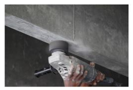
Initial surface preparation of the concrete substrate by grinding or grit blasting (where permitted).
