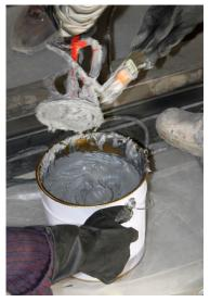
Mix the **MasterBrace ADH 4000** epoxy adhesive PTA and PTB together into a streak-free colour using a suitable slow speed mixer and mixing paddle. Ensure the sides of the tin are scrapped down and material re-mixed thoroughly.
