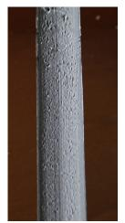
Ensure that the entire surface of the **MasterBrace LAM** is covered with the **MasterBrace ADH 4000 adhesive**. Do NOT leave any bare spots on the surface of the LAM as this will create air voids within the **LAM** application once cured.
