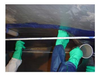
g) Allow sufficient time between the application of MasterBrace FIB material on the first coat of wet saturant and the application of the second coat of saturant. This is to allow for epoxy impregnation and is suggested at around 15 minutes (depending on ambient conditions). Any lifting or delamination that may occur during this period, must be corrected by pressing down the MasterBrace FIB Fabric using a de-foaming roller or rubber squeegee.
