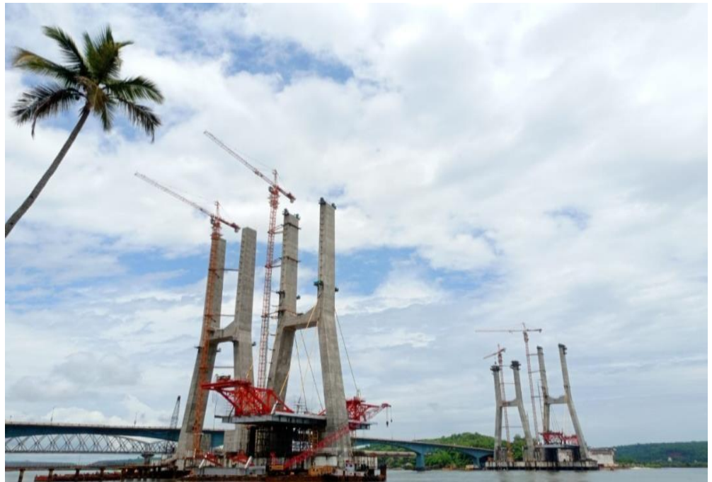
Zuari Cable Stayed Bridge, Goa, India
