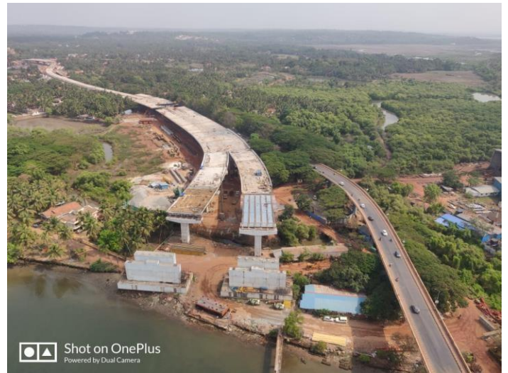
Zuari Cable Stayed Bridge, Goa, India
