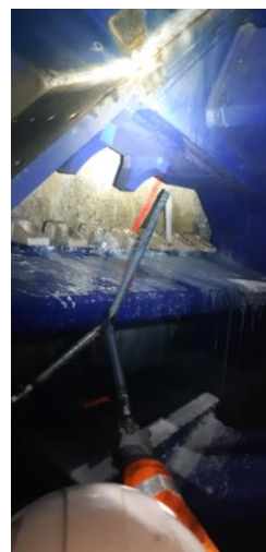
Figure 2 – Picture showing the spraying of SWA polymer from within the cutterhead
