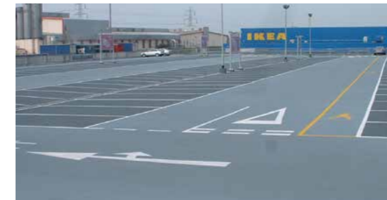
MasterSeal Traffic 2500 HD IKEA Leeds, United Kingdom
