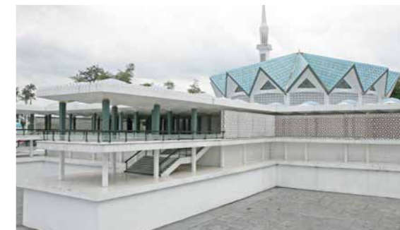
MasterSeal Roof 3500 National Mosque Kuala Lumpur, Malaysia
