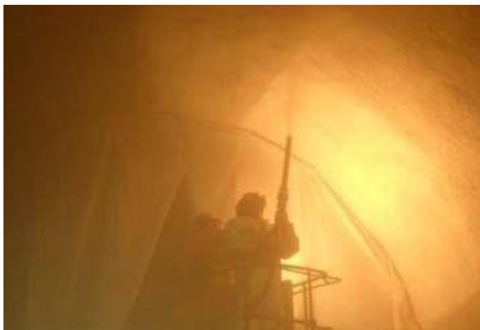
Photo: Application of shotcrete in the tunnel
