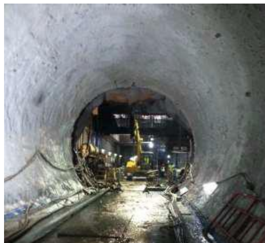
Photo: Underground tunnel of Hong Kong West Island Line
